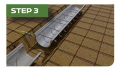
Prior to joining the flanges, apply a continuous bead of silicone along the flange to prevent leakage.
