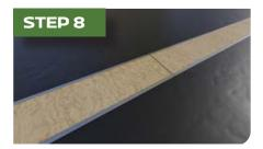
Once the first concrete pour to set has properly set, the floor slab can be completed. The use of a pencil vibrator is strongly recommended to make sure that the concrete has completely surrounded trench drain, leaving no bubbles or voids.
