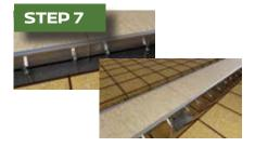
To ensure that the trench drain will not float, it is recommended that the concrete be poured in two stages. The first stage is a concrete slurry to secure the drain bodies.
