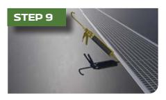
Once the concrete slab is firm, remove the plywood and place the grating on the drains. It is also recommended to apply the silicone bead between the drain top edge and concrete to avoid any water seepage between those points of contact.
