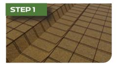
Identify the installation location of the trench drain and excavate a linear trench, allowing for room underneath and on both sides of the trench drain. Allow for a minimum of 6" of concrete surrounding the drain.
