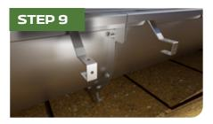
Once the concrete slab is firm, remove the plywood and place the grating on the drains. It is also recommended to apply the silicone bead between the drain top edge and concrete to avoid any water seepage between those points of contact.
