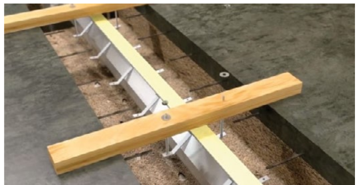
WOODEN PIECE PLACED ON THE DRAIN
