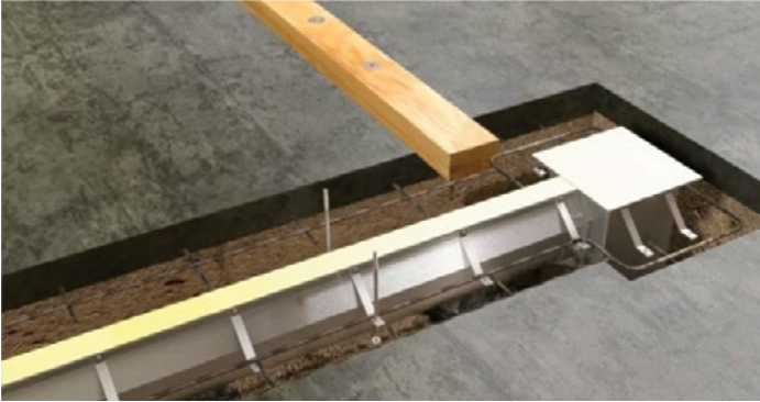
WOODEN PIECE REMOVED FROM THE DRAIN
