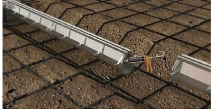
SILICON SEALANT APPLIED IN THE FLANGES BETWEEN DRAIN CONNECTIONS
