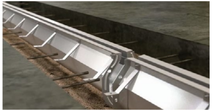
SILICON SEALANT APPLIED AND BOLTED BETWEEN ONE DRAIN FLANGES
