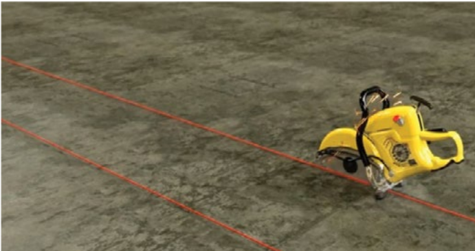
CUT THE TRENCH IN THE SLAB
