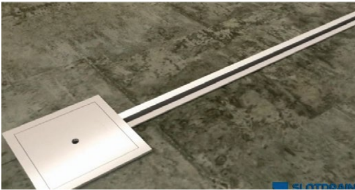
REMOVE THE DUCT TAPE FROM THE SLOT OPENING
