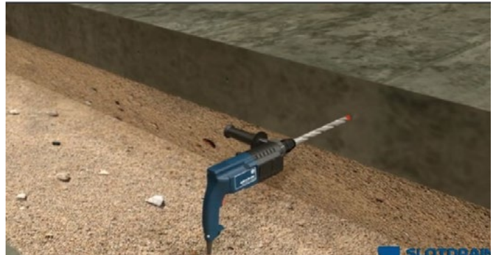
DRILL THE SIDES OF THE SLAB
