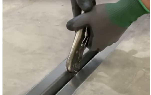
REMOVAL OF METAL TABS
