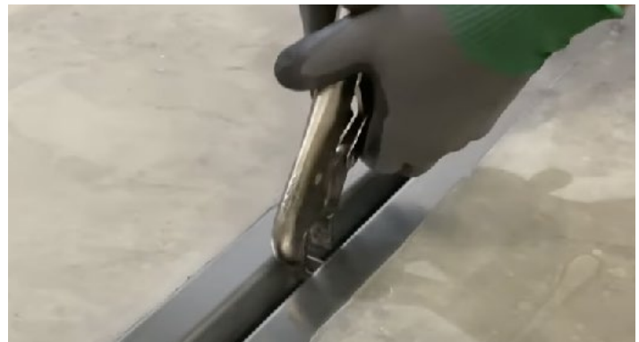
REMOVAL OF METAL TABS
